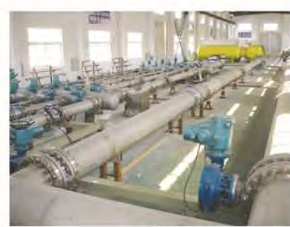
Flow Resistance Testing
